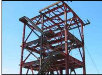
BA Silo Structure
