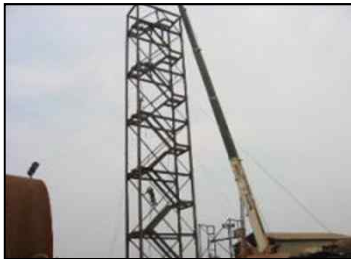
FA Silo Tower
