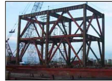
FA Silo Structure
