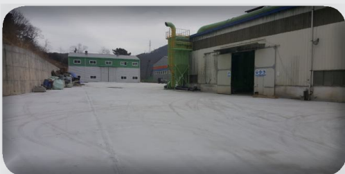
Warehouse / 2nd Foundry
