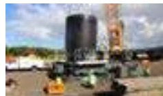
CASING OSCILLATOR
